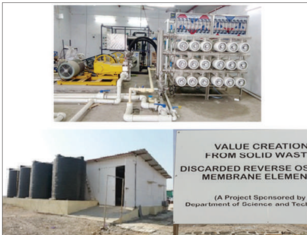
Membrane rejuvenation Pilot plant at Experimental salt farm, CSIR-CSMCRI Bhavnagar
